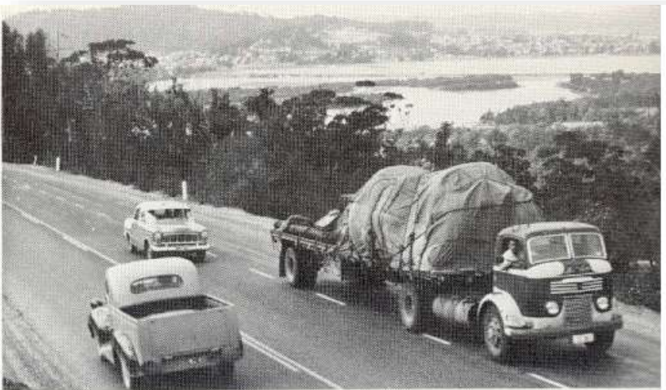
The State's first additional "climbing" lane for slow-moving vehicle was built on the Pacific Highway south of Gosford in 1954.
