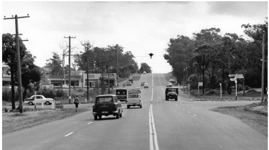
1950's Wakehurst Parkway Intersection with Blinking light above the centre of the road.
